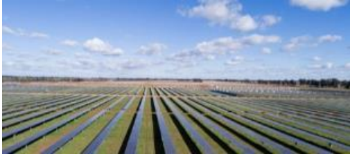
PARKES SOLAR FARM
